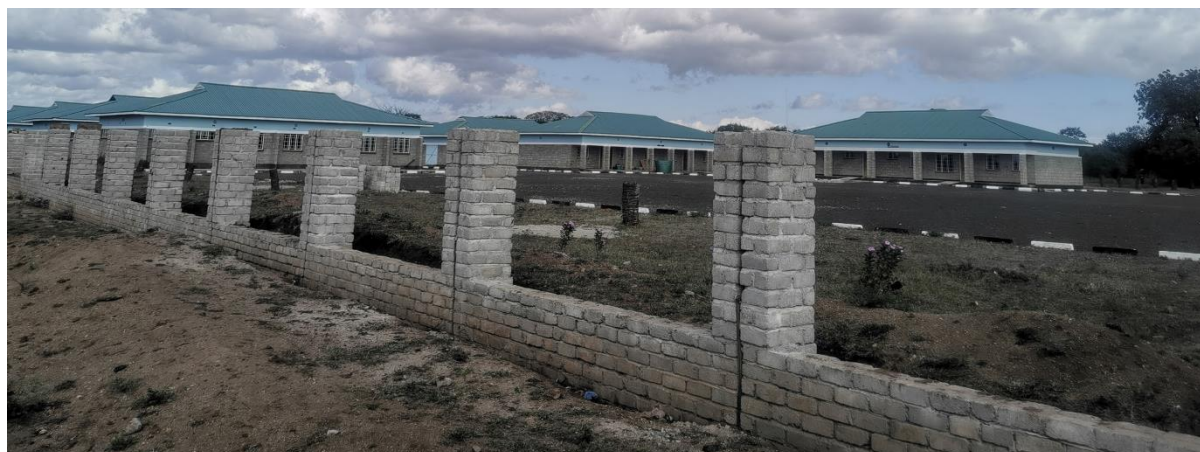
Figure 5: Shows newly constructed Ngabu Technical College (Physical Planning Department, 2022)
